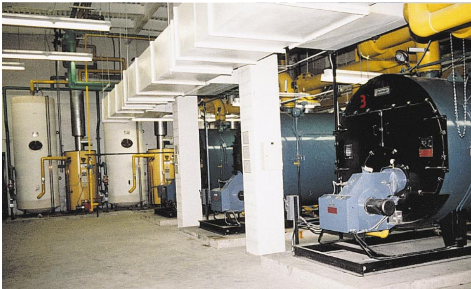
New gas-fired boiler plant. The new gas-fired domestic water heaters and storage tanks are shown at the left rear.
